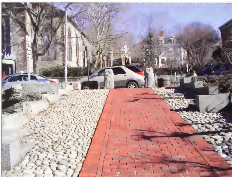
Figure 2.15 (right). The ramped eastern end of Walk F showing its cobblestone shoulders, stone retaining walls, and stone bollards, looking east with St. John's Cathedral in the background, 2008. The treatment of this walk was intended to recall the character of Church Street, which remains across North Main Street. The walk to the Old State House has a similar cobblestone shoulder. (SUNY ESF.)
